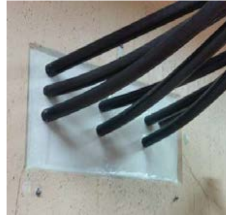
Typical sample of penetrating services with gaps above 30mm or mixed services
