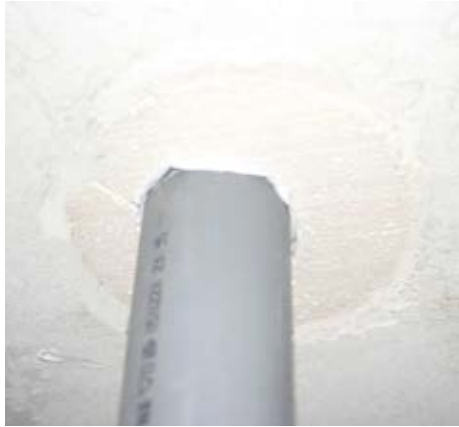
Typical sample of penetrating services with gap widths between 0 and 10mm
